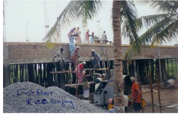
Construction Site: Second Phase
